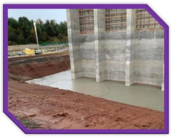
These two images show the comparison of heights from the start of works to the last pour, illustrating the 4 metres of lift and the draft angle of the excavated face.
