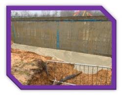
In total, at least four large voids that spanned the width of both tanks, these needed to be filled from both sides, Material was excavated in order to assess the extent of the voids or sinkholes.
