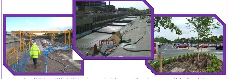
Some 28,000 m³ of 450kg/m³ highly air entrained cellular concrete (foamed concrete) provided at Gerrards Cross, . Foamed Concrete specified to reduce the loading after traditional infill material caused the tunnel to collapse onto the railway.
