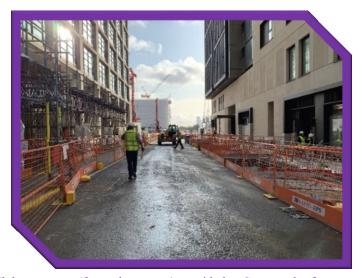
Some 30,000 m<sup>3</sup> Sub 500kg/m<sup>3</sup> highly air entrained cellular concrete (foamed concrete) provided at Canary wharf, London. Foamed Concrete specified to reduce the loading and encapsulate all new services and drains /sewers. Placed in 500mm deep layers.
